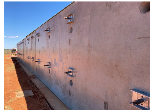
View of completed panel placement and tie rod installation
